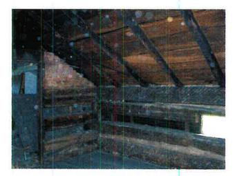
▼ This view of the wall looking into the braced timber frame part of the house shows the flu vent for a stove and the brick fill that was used above the top course of logs. The floor of the second story was wide poplar planks of various widths.
