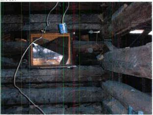
▼ The rafters consist of logs hewn on only one side. The wide roof planks were characteristic of early and mid 1800's construction. The original doorframe shown here was pegged as were the window and doorframes throughout the log home. This construction was also typical of early and mid 1800's construction.
