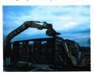
▼ Straps were tied to the ends of the logs and they were chained in the middle and lapped over the teeth of the crane's bucket. Using this method, they were easily lifted onto the trailer.
