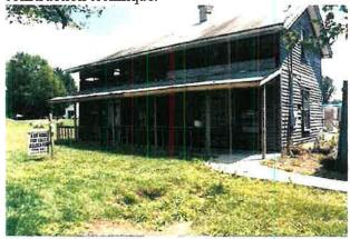
▼ The log home was built in the traditional "single pen" construction, which consisted of a single room on the first floor. This log home, located near the center of the City of Green, underwent many changes through the years. In fact, it was changed so much that it was no longer recognizable as a log home.
